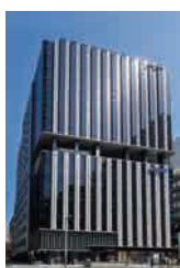
PILOT Corporation head office
