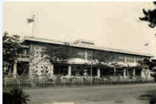
Construction of the Hiratsuka General Plant
